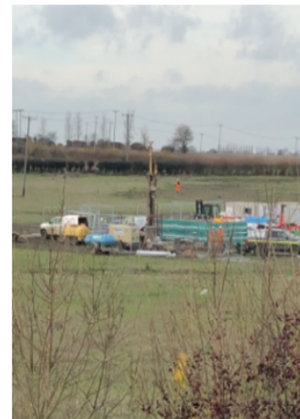
North Cutting Pump Test Bore Hole under construction showing water escape 24/11/20
