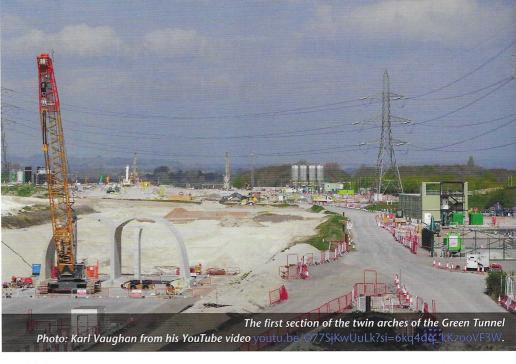
2019. The term 'gap' refers to the constricted area south of Wendover containing the A413, the Chiltern Railway line, the National Grid and a range of underground utilities. The 2017 High Speed Rail Act defined that this part of the line would be through a 'cut and cover' tunnel past Wendover, going under Ellesborough Road. It also specified that six houses would need to be demolished to enable the green tunnel to be constructed.
