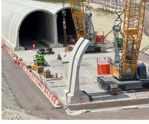
for similar tunnels on the TGV railway in France. Each segment is made up of five parts which fit together in a weight-bearing pair of arches, without any need for mortar or additional concrete to hold them in place during construction. They arrive by road, as and when they are needed, from the manufacturing plant in Derbyshire. The Ellesborough Road diversion's Bailey bridge is a useful vantage point to watch them being put together using a 1,200-tonne crane.
