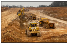
Cutting works near Great Missenden
