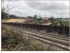
Sheet piled retaining wall
