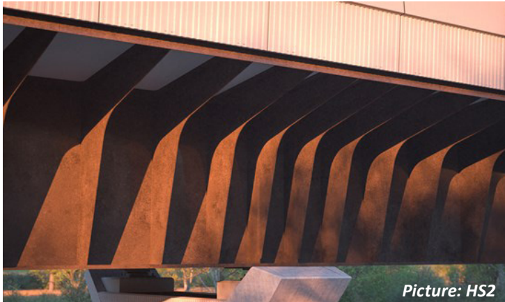
An artist's impression of the viaduct showing a close-up of the weathered steel box girder, support fins and the bottom part of the 1.8m high textured concrete cladding
