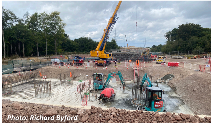
Each of the ‘hammerhead’-topped upright piers sits on a thick concrete foundation, supported by reinforced-concrete bored-piles sunk into the hard ground 49 metres below
