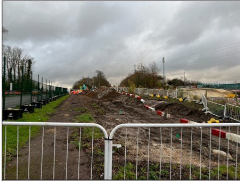
Viaduct excavation site beside the A413 at Small Dean.
