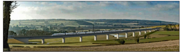
Artist's impression of Wendover Dean viaduct for HS2 Ltd, in fields east of the A413, passing over Bowood Lane, see also https://chilternsociety.org.uk/hs2-photo-diary/ .
