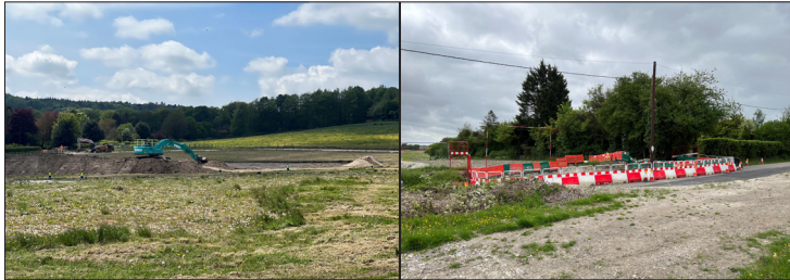
Photos of the road excavation and water main works
