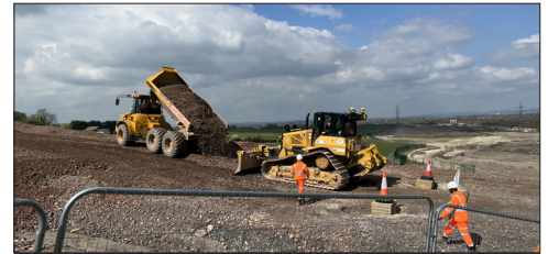
Building relief embankment Ellesborough Road
