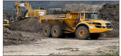
Topsoil stripping Ellesborough Road field
