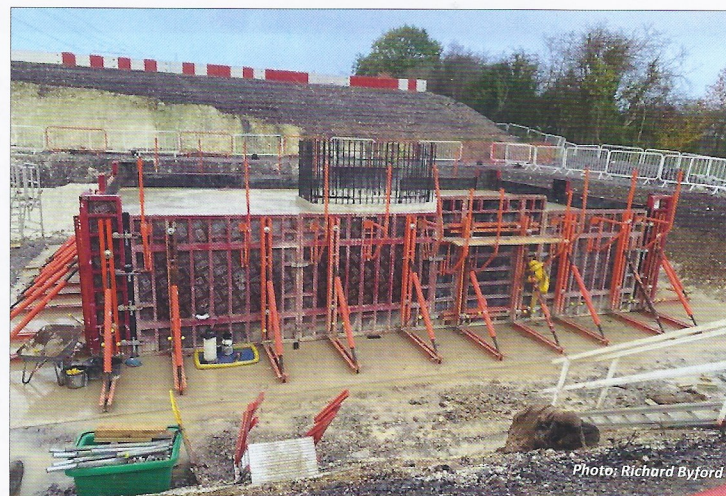
A below-ground level look at a typical foundation slab. These are made of poured concrete on top of an array of piles which often go down tens of metres.
