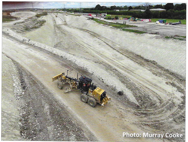
One of the graders employed to maintain the haul road in serviceable condition
