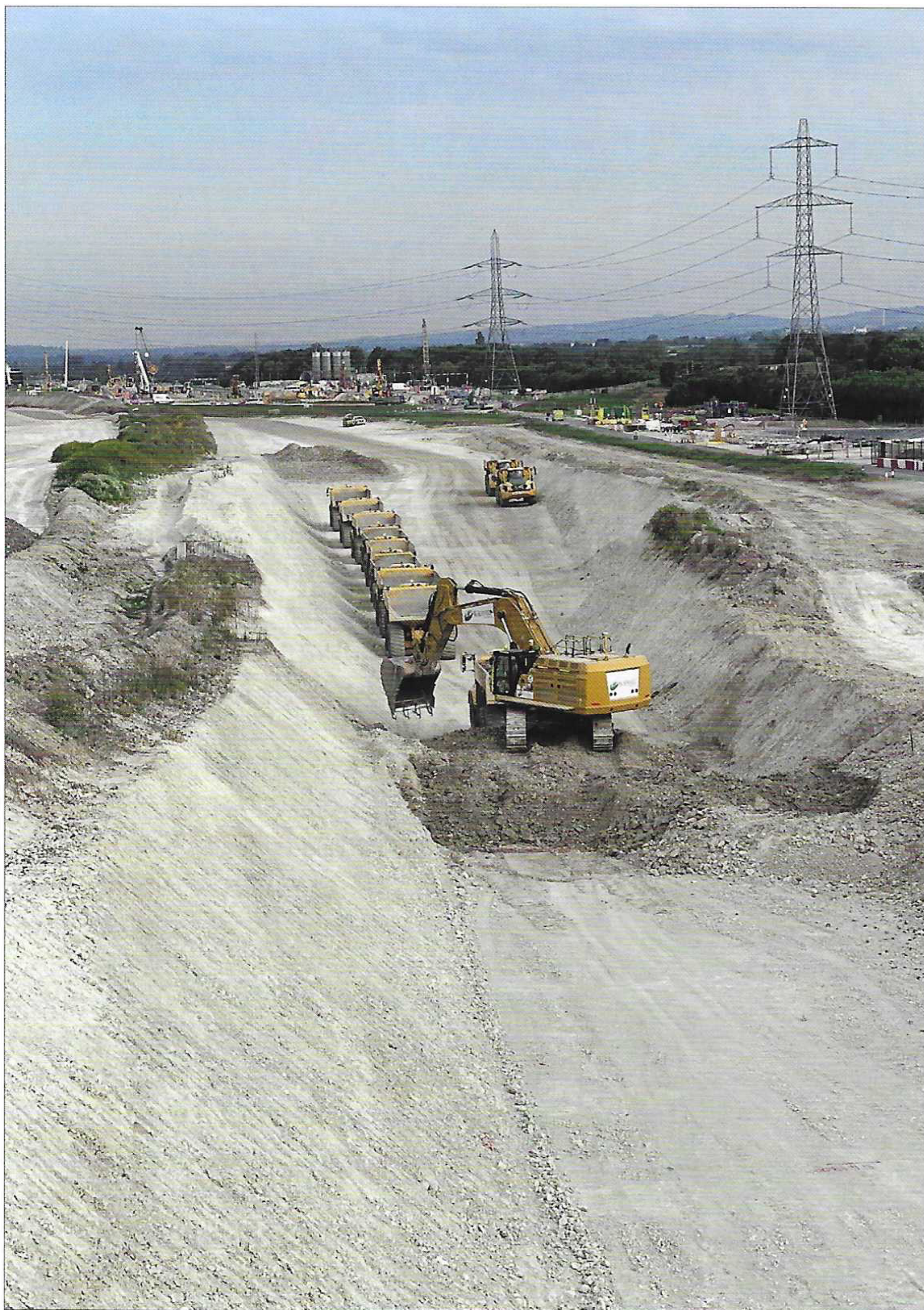
Fleet of dump trucks on the haul road north of Ellesborough Road
