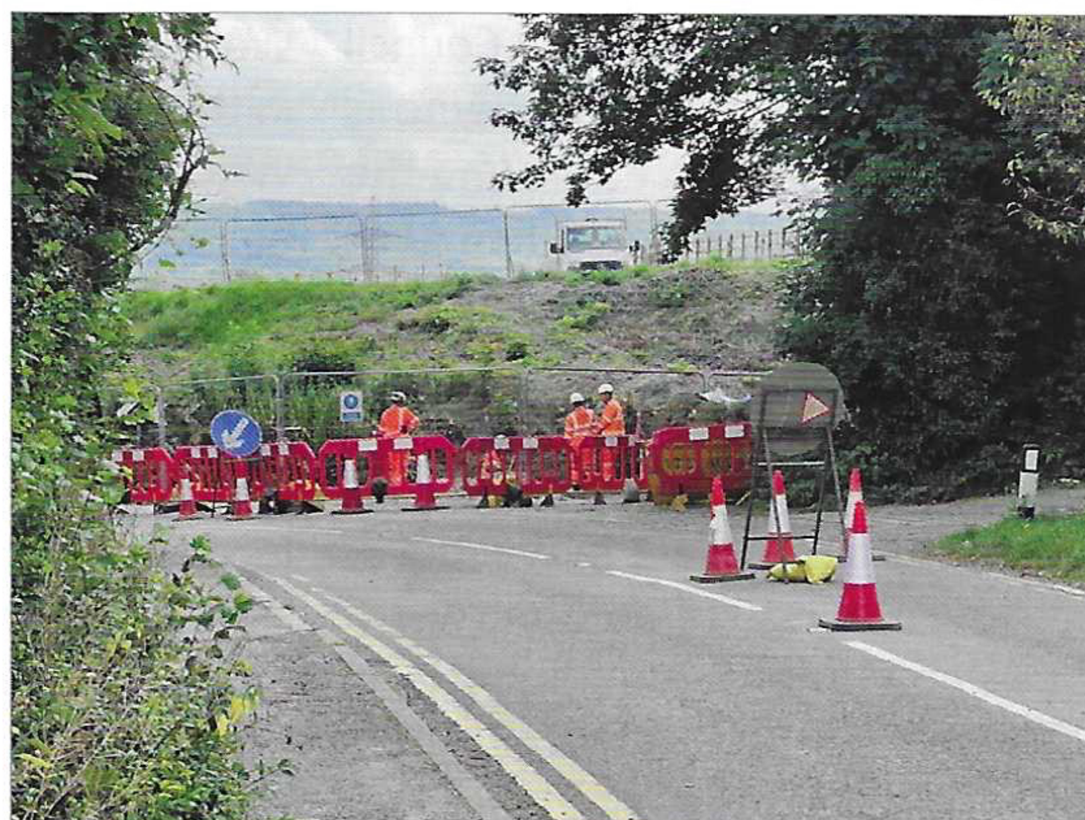
Building the new link road junction at Ellesborough Road
