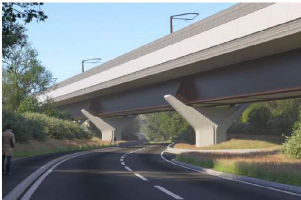
Small Dean Viaduct - A413 London Road view
